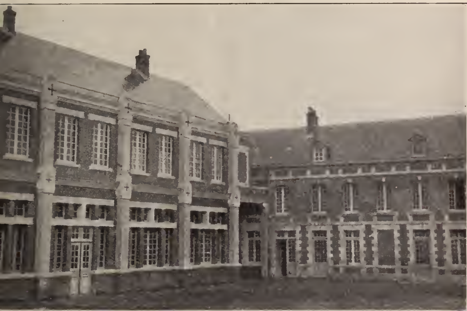
THE SPLENDID NEW PLANT OF THE FRATERNITÉ AT ST. QUENTIN
